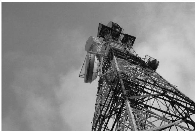
Figure 2.2 Microwave towers Microwaves are beamed from tower to tower.
